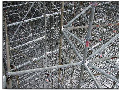
Figure 7.41 Even before the broadcast compound takes shape most venues needed spectator facilities constructed. Here is some of the massive assemblage of scaffolding that was required for spectator seating at the Alpine skiing venue. (Source: Chadwick Wachs)
