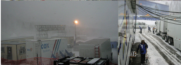
Figure 7.46 A key technical part of every venue was the technical operations center (TOC). All video, audio, communications and computer data at the venue funneled through the equipment in this office trailer. Half the production trucks used at Salt Lake produced and processed the video as digital data. A few of the trucks also processed the audio as digital data. Trucks that still worked in the analog domain temporarily installed equipment that converted their analog outputs to digital. The trucks also installed equipment that would embed up to eight channels of audio into the horizontal interval of the video data. Thus Vanda went from the trucks to the TOC as digital data. Inside the TOC the combined Vanda, now a 270Mb/s data stream (SMPTE 259A) was wrapped in OC-48 SONET frames and put onto the SONET ring that the venue was connected to. Each ring could handle nine full bit rate digital Vandas. Another important function of the TOC is to monitor the quality of the signals leaving its venue. (Source: Jason Taubman)
